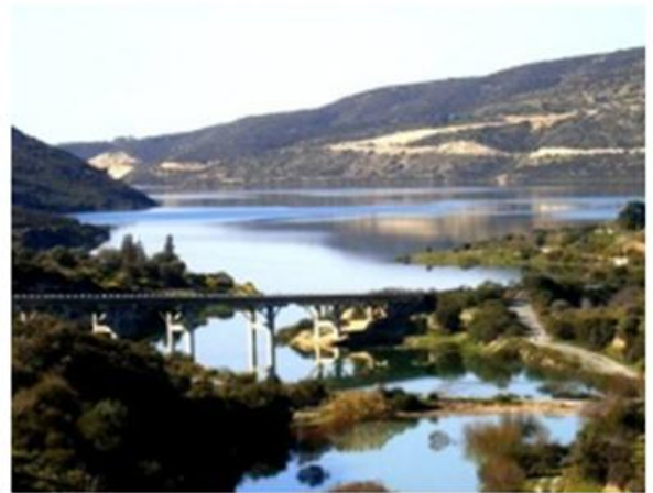
Image 3: The Kouris dam is the largest dam in Cyprus. Three rivers end up in this dam: the river Kouris, the river Limnatis and the river Krios. It's placed in the district of Limassol.
